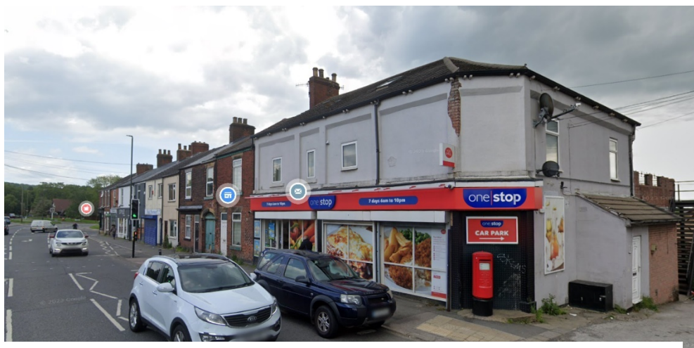
Existing streetscene – terrace row facing north east and south west
